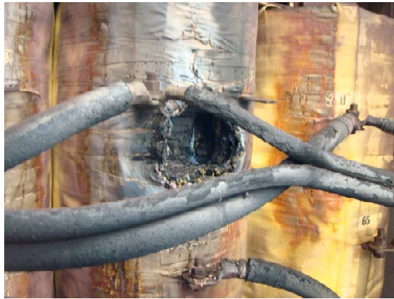
Figure 11. 4.16 kV Reduced Voltage Auto Transformer Starter Failure Due to Breaker Switching Transients
