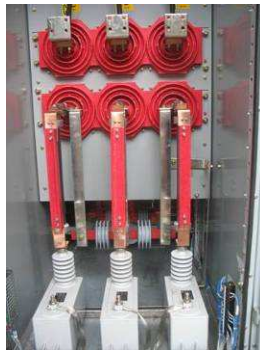
Figure 21. Snubber for Metal Enclosed 13.8 kV Vacuum Breaker
