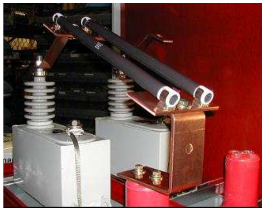
Figure 17. 15 kV Snubber Mounted Above the Transformer
