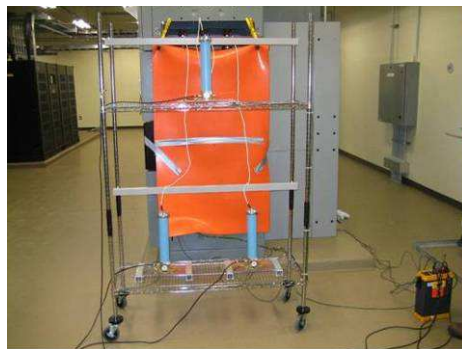
Figure 22. Snubber Performance Measurement Setup for 15 kV Transformer Using High Bandwidth Voltage Dividers
