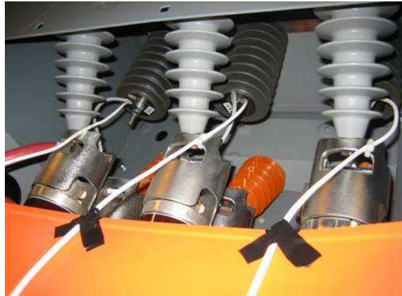
Figure 23. Voltage Divider Connections at 18 kV Surge Arrester on Transformer Primary Bushing
